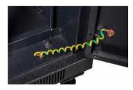
Elements of the cabinet's structure are equipped with grounding cables, which allows it to be connected to the building's grounding system, ensuring safe and proper operation of the devices installed inside.
